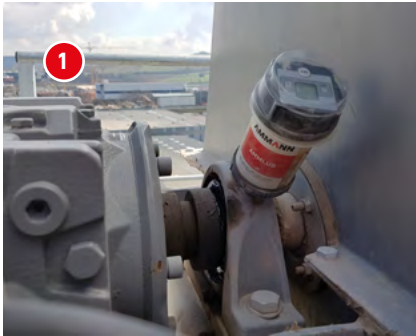
HOT AND FILLER ELEVATOR
